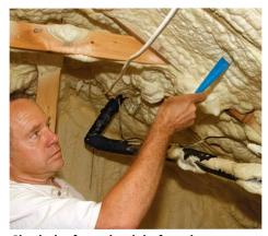
Check the foam depth before the crew leaves. Once the spray foam expands, poke it in various areas with wire to measure how deep it is. A depth gauge made of wire and blue painter's tape confirms the foam depth. The wire is so thin that the hole it leaves will not affect the foam's performance.
