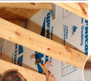
Isolate conditioned space. Tack OSB, Thermo-Sheath (www.fibreconverters.com), or Thermo-ply between trusses where they overhang an exterior wall. Canned spray foam is a good way to seal the sheathing in place.
