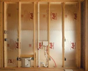
Some interior walls might need sheathing. Spray foam is most often applied against plywood or OSB sheathing. In some cases, such as this laundry-room wall, which will be sprayed for sound-deadening, you need to install a substrate for the foam. Here, Thermoply, an inexpensive cardboardlike material, is nailed to the studs to carry the spray foam (www.covalence coatedproducts.com). Later, drywall will be added over the Thermo-ply.
