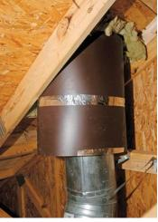
Wrap stovepipes to maintain insulation clearances. To create the clearance specified by the stovepipe manufacturer, wrap two bands of 12-in. aluminum flashing around the pipe. After installing the lower band, cut the upper band to the roof's pitch, and attach it to the rafters or truss with roofing nails. Aluminum tape holds the two together. Fireproof rock-wool insulation or fire caulk fills the remaining gaps.
