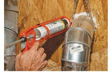
**Seal penetrations with caulk.** Expanding spray-foam insulation will find its way through any crevices larger than ½ in. Caulk around pipe penetrations before the spray foam arrives to keep it from seeping onto the siding.
