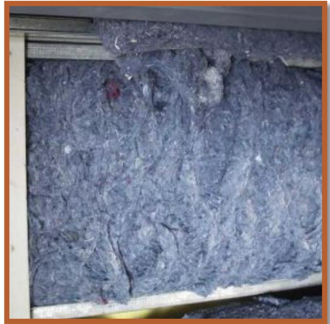
Blue-jean insulation doesn't cut easily, it's difficult to install, and it doesn't expand well. It's just not that green.
