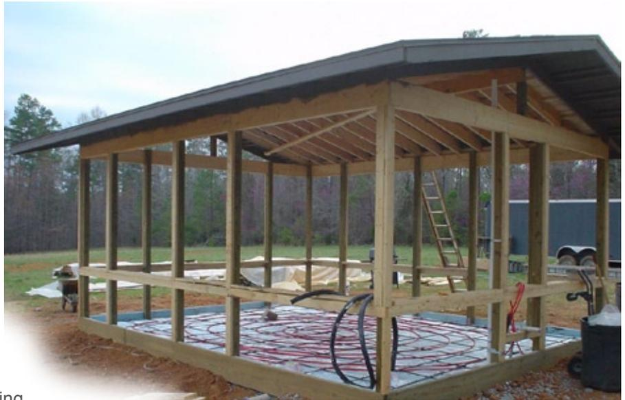
Construction starts by digging and pouring 22"x22"x10' pier footings at each post location. Then the posts are set, braced and anchored to their footings.
