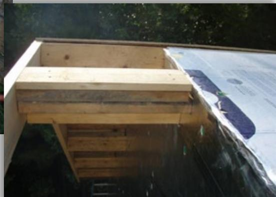
A 2 3/4" wide steel flashing combined with a treated 1x4 and soil treatment keep the termites and insects out of the structure. At the top the wall foam is foil-taped to the foam on the roof. The structural roof outriggers are packed up 2 1/4" to accommodate 1" of ceiling planking, a 1/2 inch airspace between the ceiling and the foam, and 3/4" of foil faced foam with the shiny side down. On top of this will go 1/2" OSB and roof shingles.
