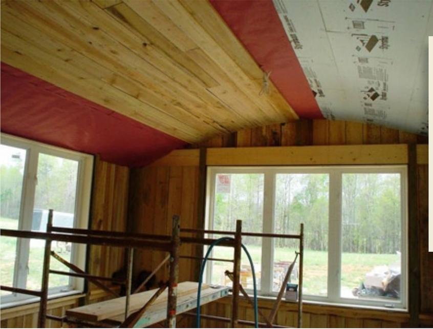
The interior got planked with a curved ceiling with both fiberglass and Styrofoam insulation. The red rosen paper is used so when the rough sawn lumber shrinks the blue foam will not be visible. The paper ages to a light brown over time.
