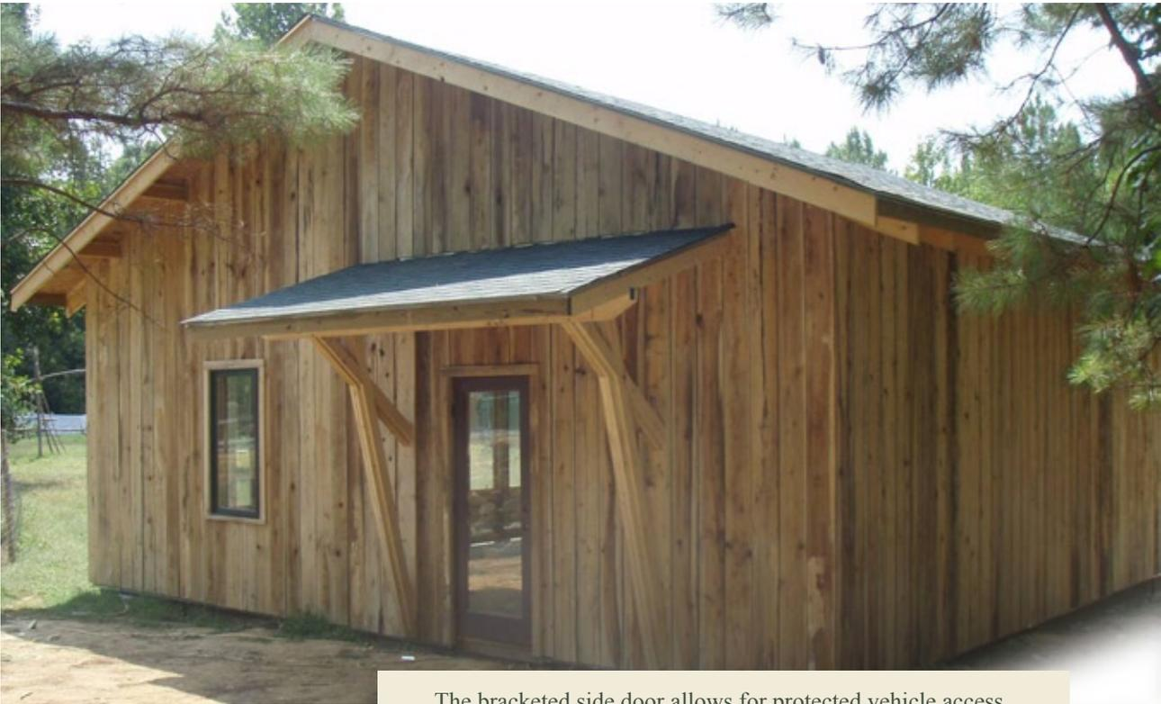
The bracketed side door allows for protected vehicle access for unloading musical gear.
