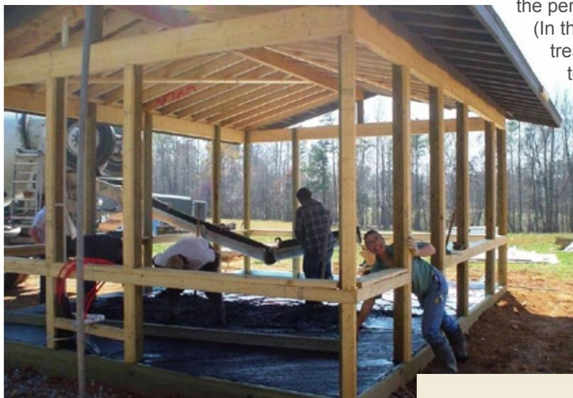
Temporary 2x10 or 2x12 concrete forms are set around the perimeter at this point if you are pouring a slab floor. (In this case, with a radiant floor, we used permanent treated form wood and tacked Styrofoam to the inside to prevent a cold edge on our heated slab.)
