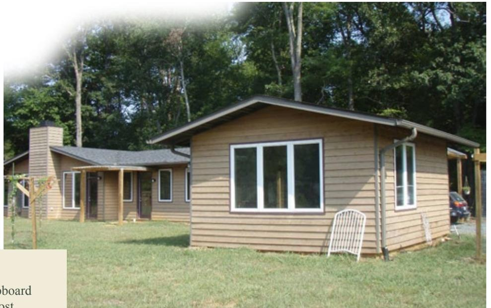
The exterior of got cedar clapboard siding to match the house. Most people associate pole barns with vertical board and batten siding which is the most common exterior for these structures but any siding can be applied.
